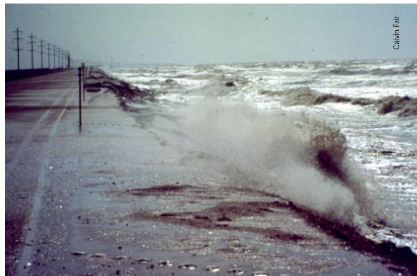
Highway 82, the only east-west highway in lower southwestern Louisiana. Once set back from the Gulf, it is now in danger of being breached. The chenier highway rests on the last ridge between the Gulf and a vast marsh plain.
